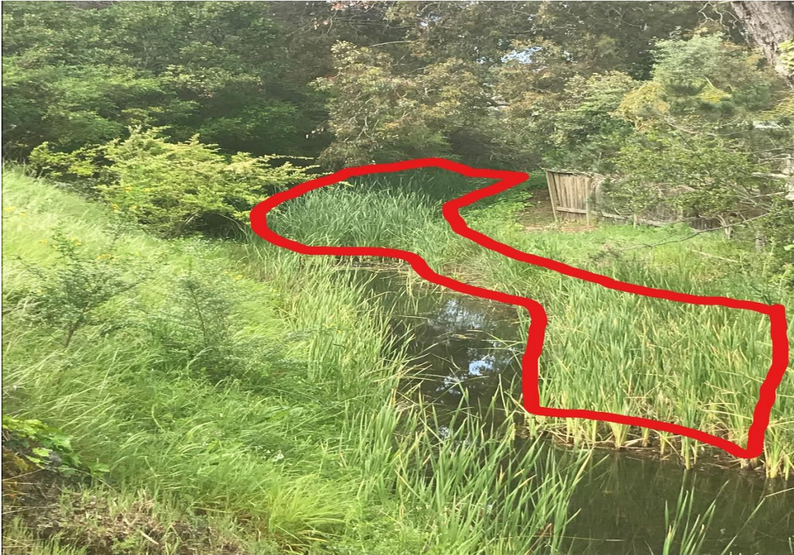
4-EAST-1 DOWNSTREAM (DS) Cecilia Way Culvert Bridge
