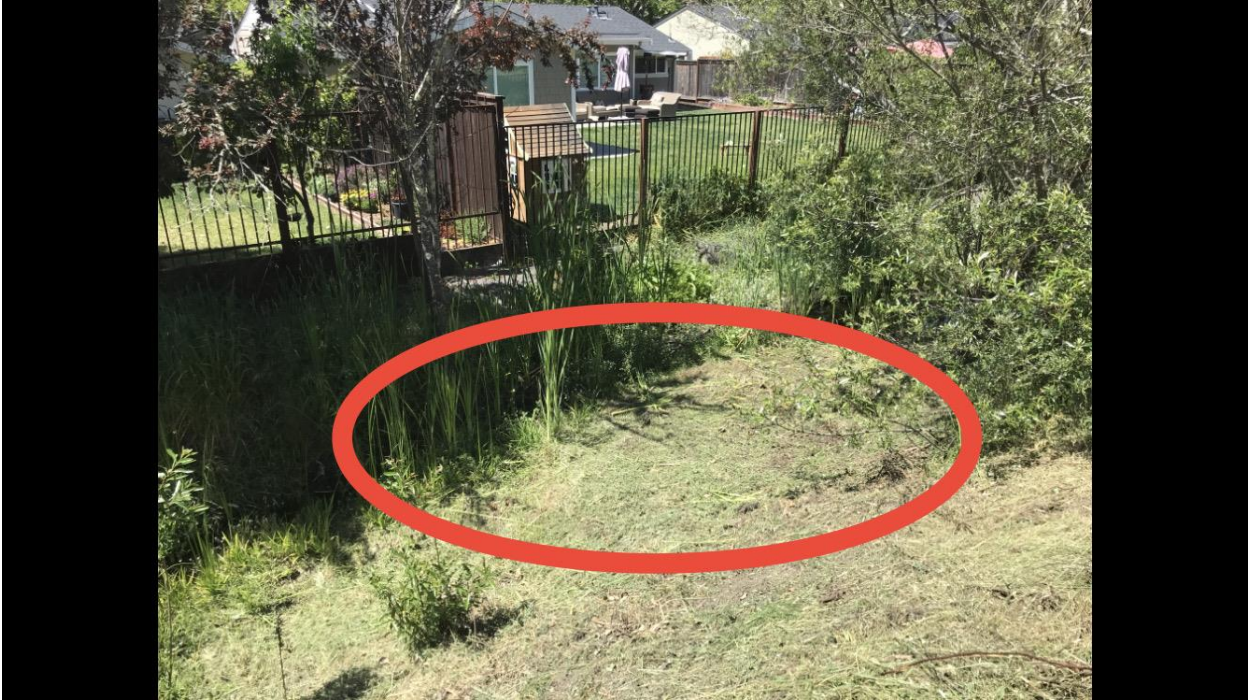
4-EAST-2 UPSTREAM (US) Cecilia Way Culvert Bridge
