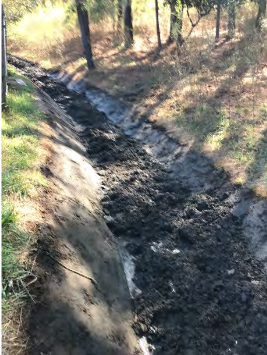
Nyhan Creek West Fork - Tam Valley Elementary School (3-NYH-2) Pre-project
