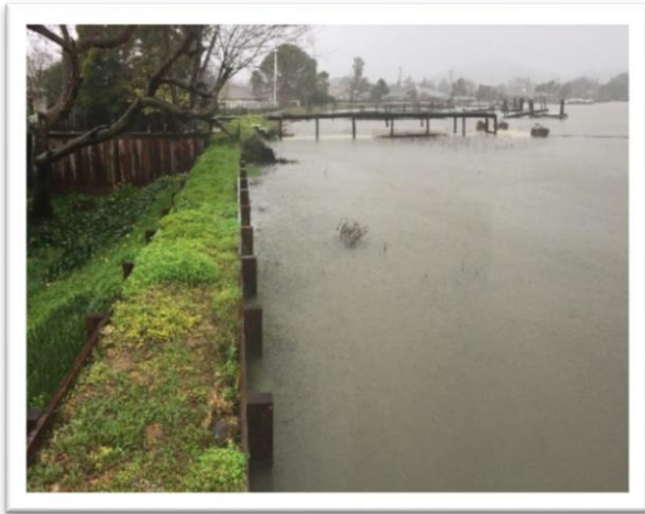
Above: Example TRB recently rebuilt and held back tides in 2017. Tides this high occur every year.
