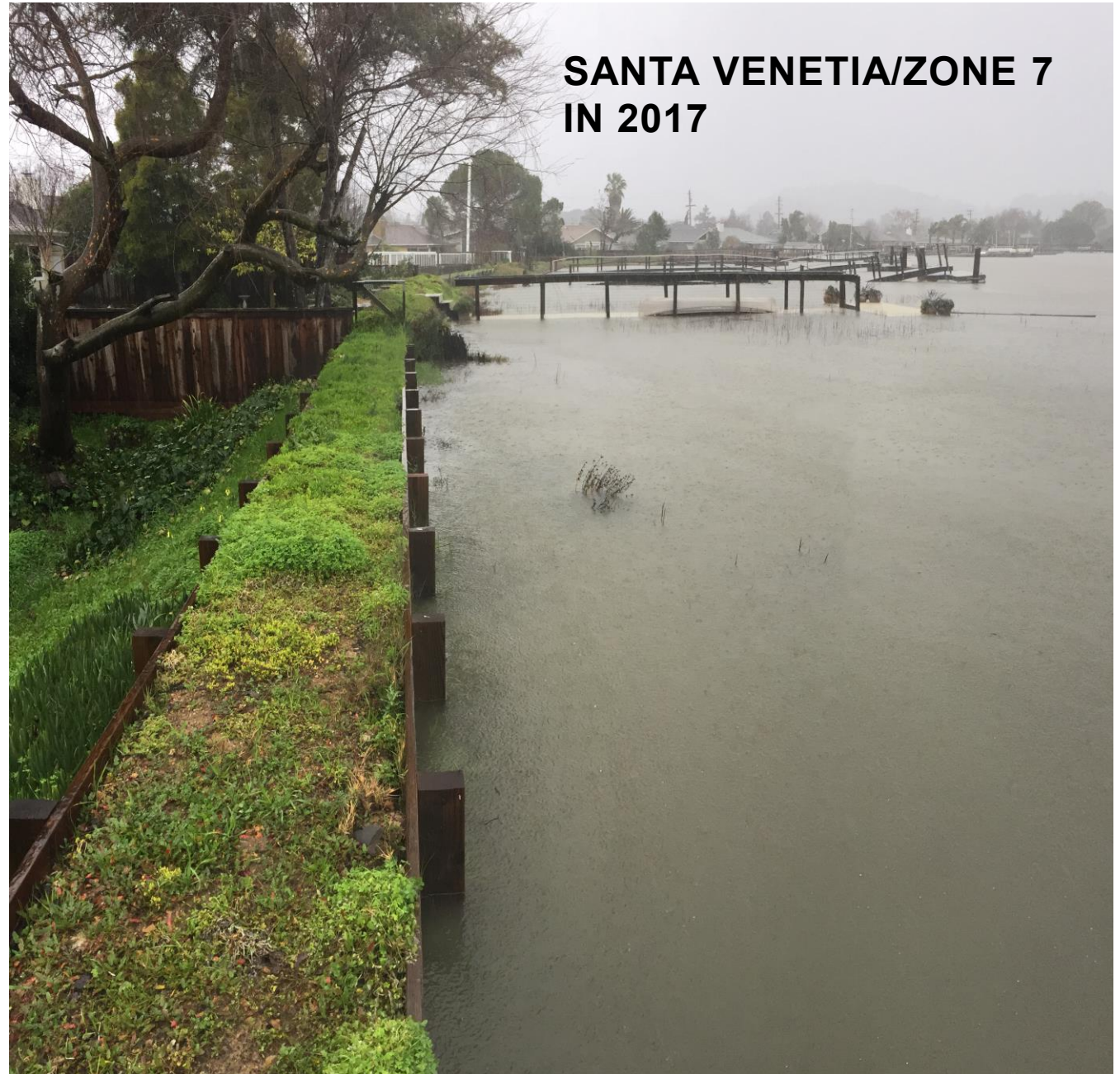
King Tide, Santa Venetia timber-reinforced berm January 10, 2017 (Photo Credit: DPW)
