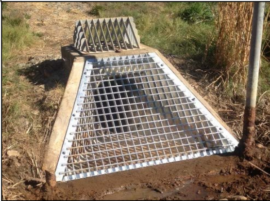
New trash rack grate at Pump Station 4
