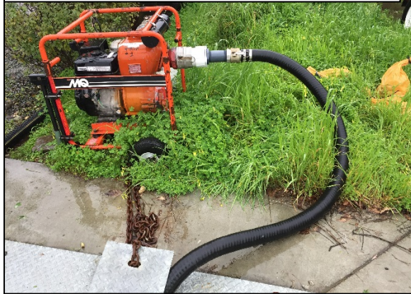
4-inch portable pump on Estancia Way
