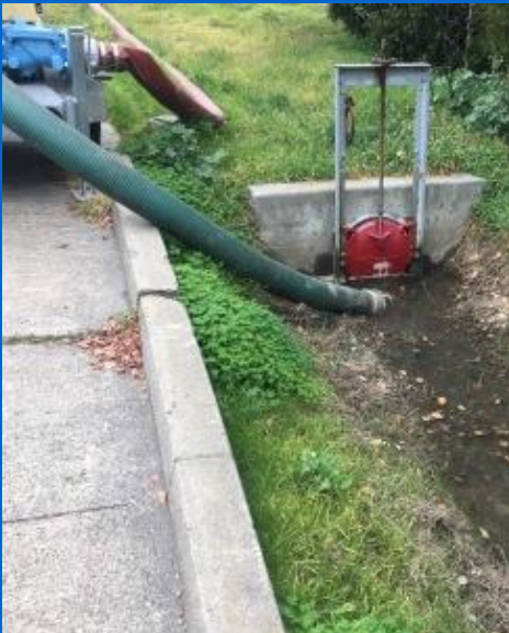
A Tideflex check valve will be inserted behind the red slide gate shown above. This will help keep tide water from entering the ditch and reduce the need for manual operation of this facility. Estimated cost is $5,800.
