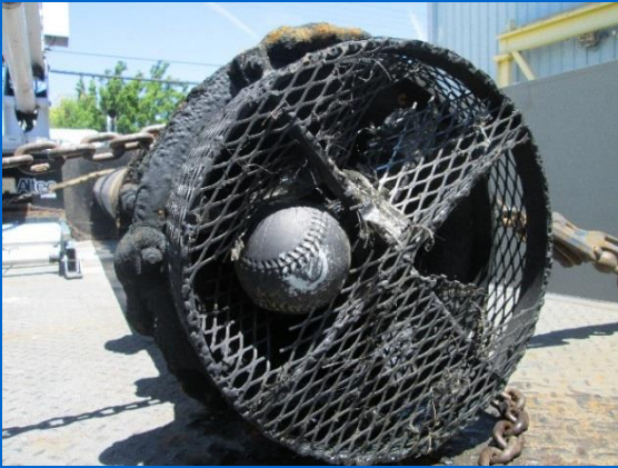
Pump Station 2 grate before annual maintenance
