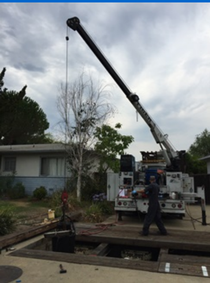
Removal of pump with crane
