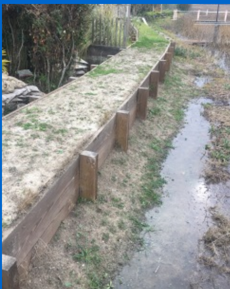
Existing Timber-Reinforced Berm:
