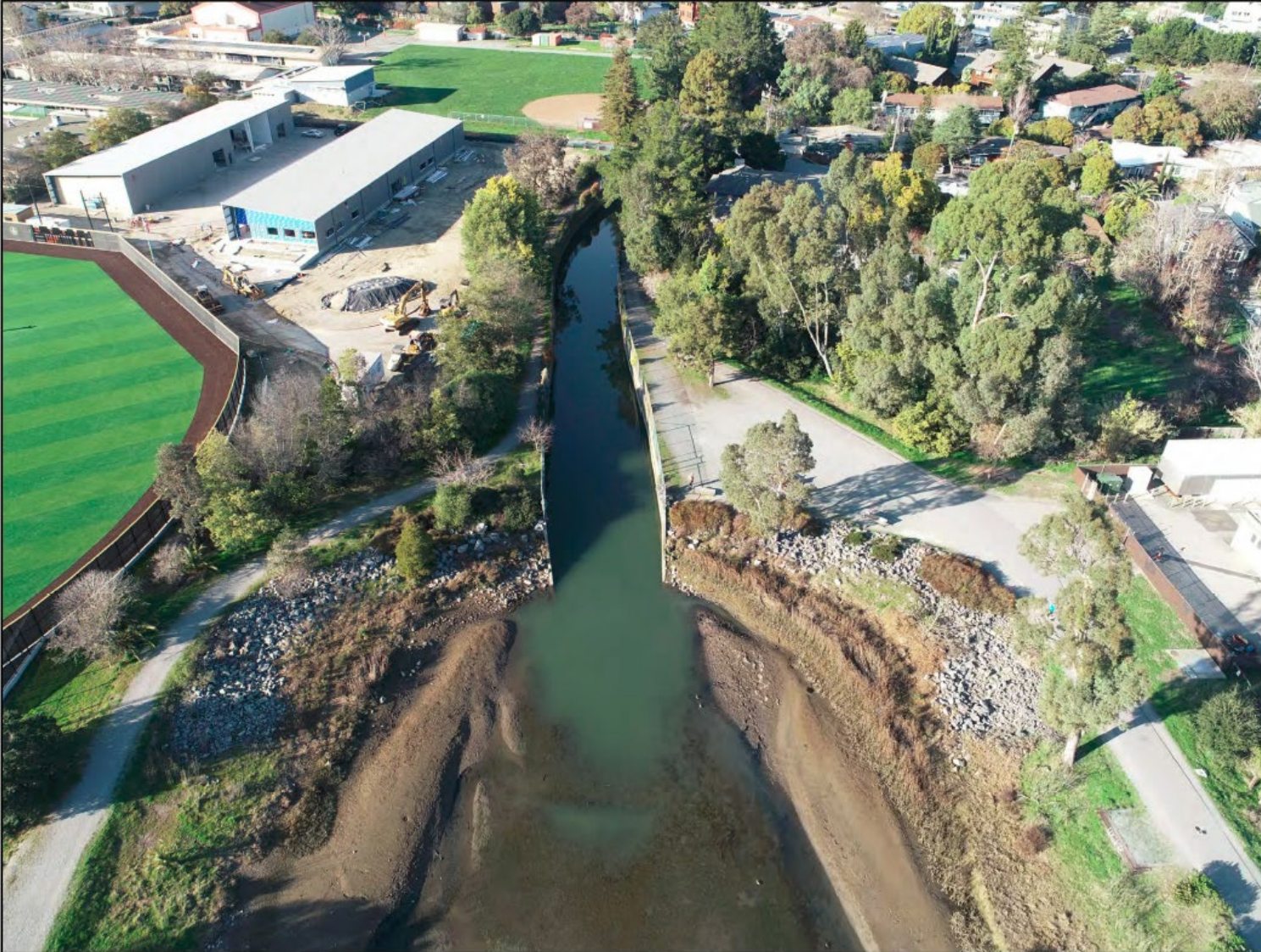
Figure 3.1-20 Existing View of Lower College of Marin Concrete Channel Removal, Unit 2
