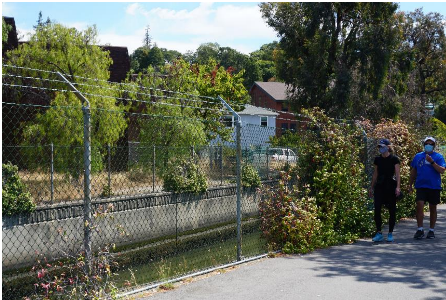
Figure 3.1-17 KOP 3: Existing View of Floodwall Location, Unit 2
