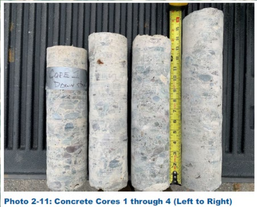
Photo 2-11: Concrete Cores 1 through 4 (Left to Right)
