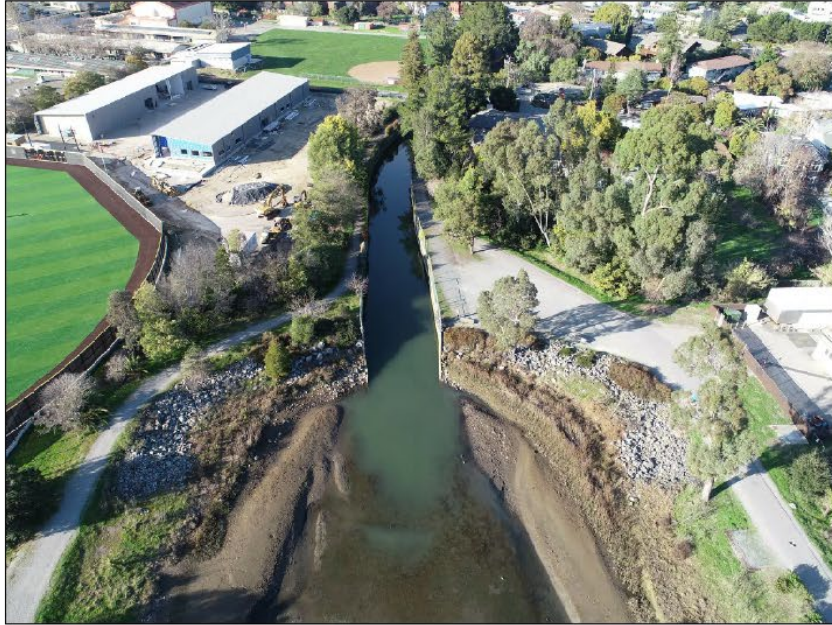
EXISTING CONDITIONS DATE OF FLIGHT: 5 FEB 2019 AT LOW TIDE (-0.3') (SEDIMENTATION DOWNSTREAM PREVENTS TIDE LEVEL FROM REDUCING BELOW 1.7' IN CONCRETE CHANNEL.)
