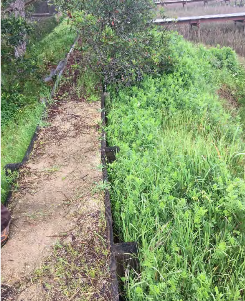
Typical section of TRB to be replaced, surrounded by upland vegetation (4/2/19)
