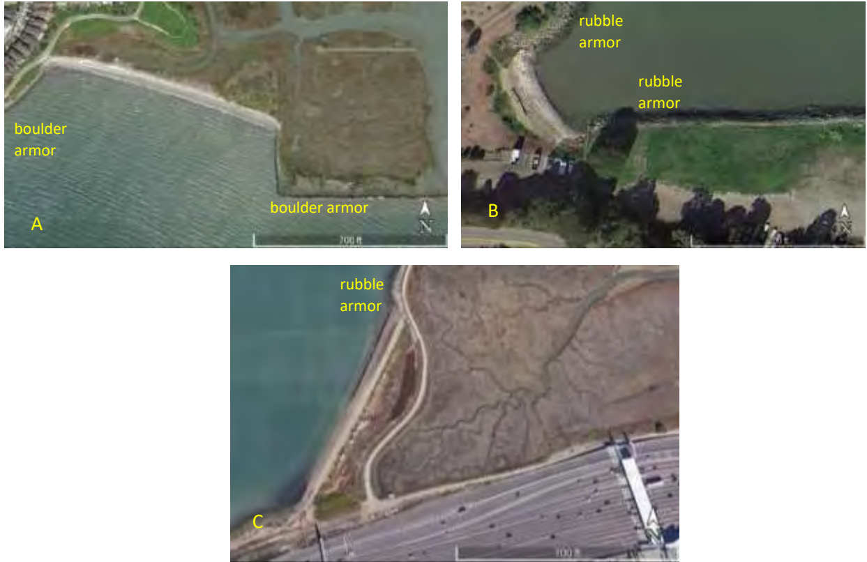
Figure 16. Examples of stable swash-aligned sand beach plan forms in artificial San Francisco Bay shores. Swash-aligned beaches naturally formed in embayments between rock-armored artificial fill headlands or fills, San Francisco Bay. (A) Marina Bay barrier tombolo (coarse sand), Richmond, showing shore-parallel wave crests along the beach, and oblique waves along the rock-armored “headlands”. (B) Starkweather Shoreline Park Beach (medium sand), Francisco Boulevard, San Rafael. (C) Radio Beach, Oakland. Images: Google Earth.
