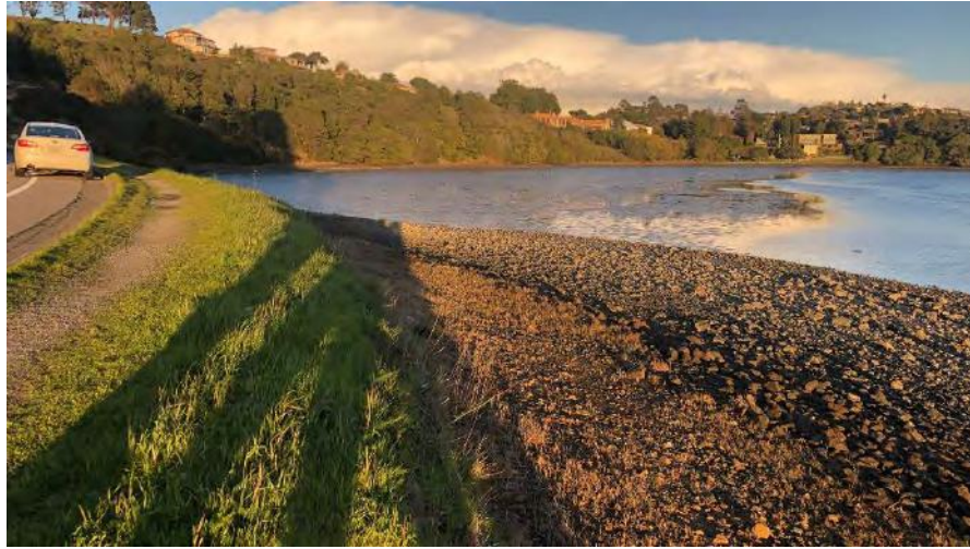
Figure 76: Top of the vertical bank near the road and bike trail at the edge of Seminary Drive. Note the existing cobble intertidal seabed extending from the base of the vertical bank. The photo was taken at mean sea level.
