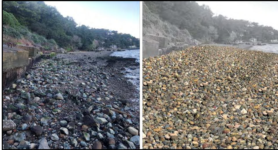
Figure 45: Intertidal area in front of the boat ramp during low tide (left) compared with a rendition of what that area would look like after placement of the bottom layer of cobble and gravel for design 1. This figure shows the material placed against the existing concrete blocks which could be left or removed, and another method of slope stabilization, for gravity slumping problems, installed.
