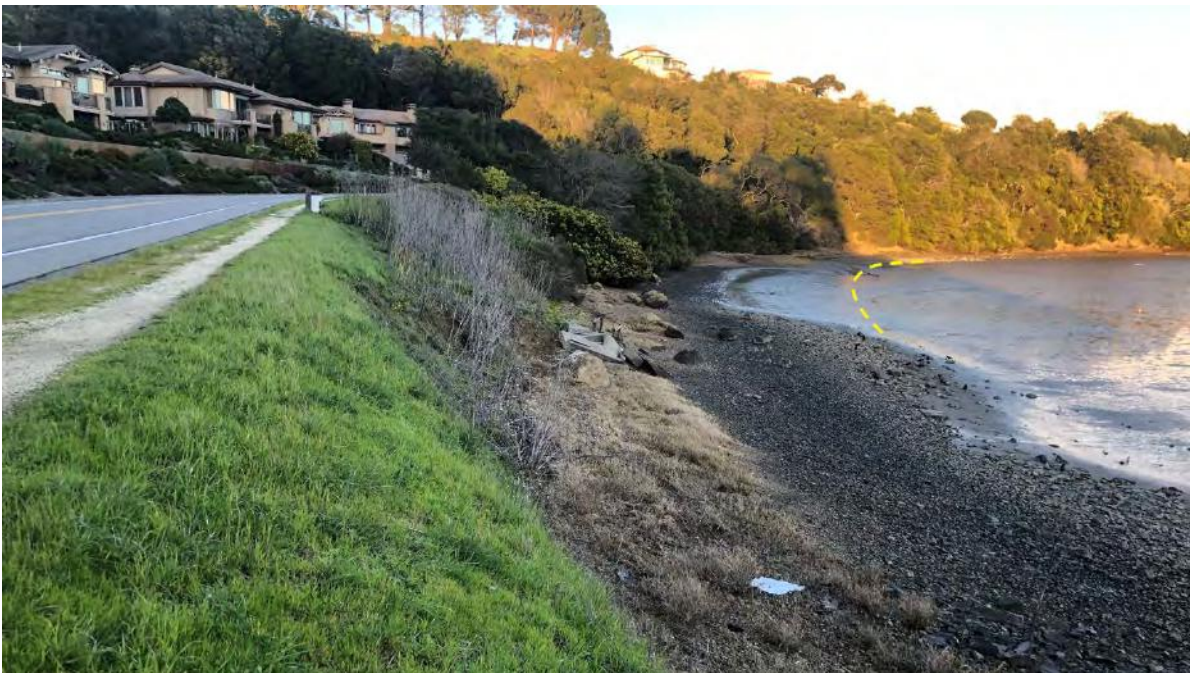
Figure 77: Top of the vertical bank near the road and bike trail at the edge of Seminary Drive. Note the existing cobble intertidal seabed extending from the base of the vertical bank. The photo was taken at mean sea level. The dotted yellow line shows where the proposed beach would blend into the existing downdrift beach. This downdrift beach would receive sand over the years effectively naturally widening the beach along the trees in that location and increasing the recreational benefits as well.
