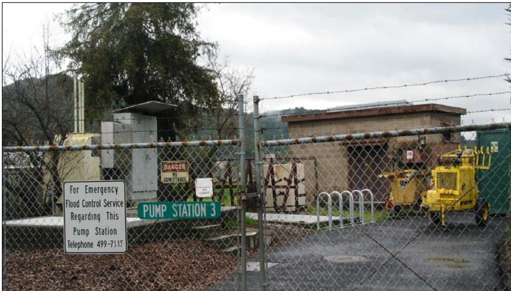
Figure 2.2. Housing Facility of Pump Station No. 3
