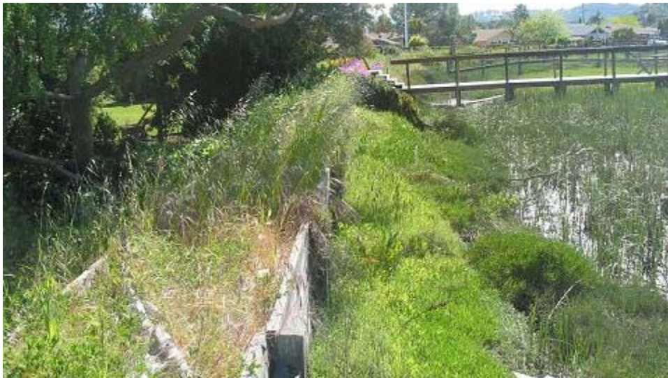
Figure 2-9. Example 2: Redwood Flood Wall/Planter Box on Top of the Earthen Levee
