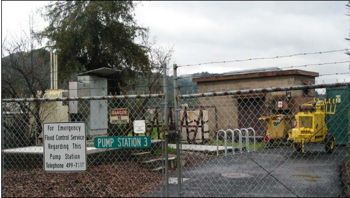
Figure 5. Housing Facility of Pump Station No. 3
