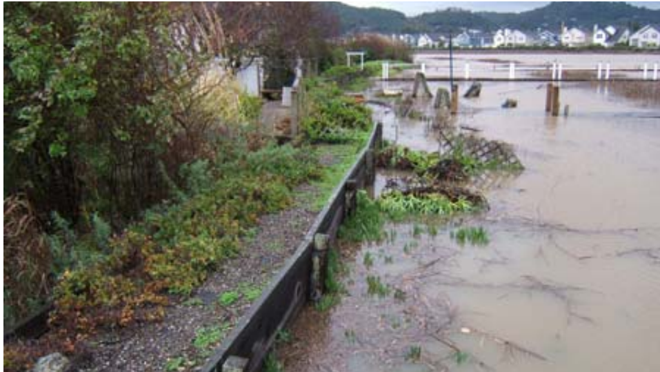
Figure 2-8. Example 1: Redwood Flood Wall/Planter Box on Top of the Earthen Levee
