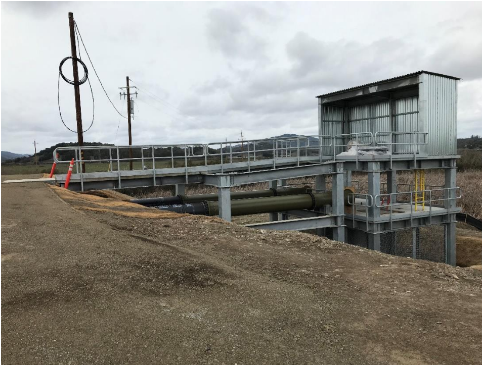
Newly constructed Simmons Slough Pump Station structure
