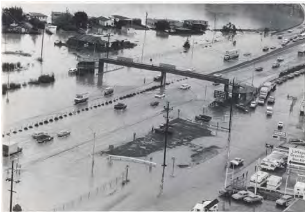
Historic Flood on US Highway 101 and fronting marshes. Larkspur. Credit: Marin DPW
