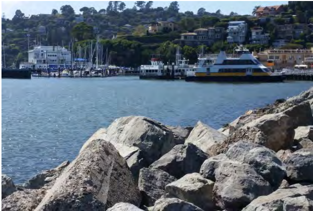
Tiburon revetment looking to Corinthian Marina and Tiburon Ferry Terminal, 2016. Credit: BVB Consulting LLC
