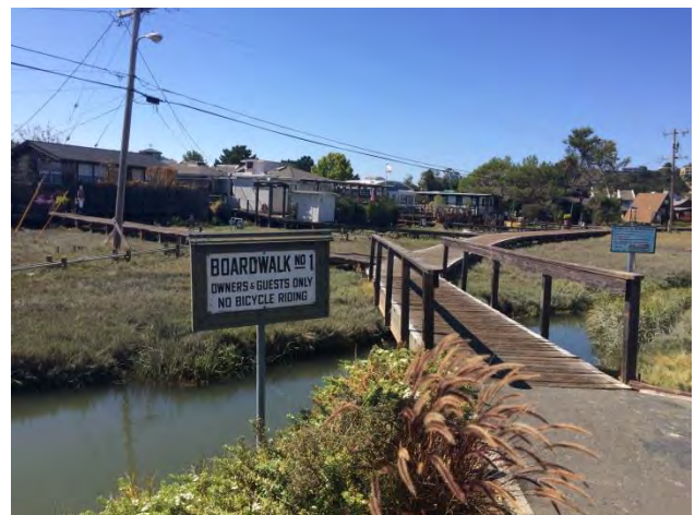
Larkspur's Boardwalk #1 with canal homes accessed via boardwalks. Credit: Marin County CDA
