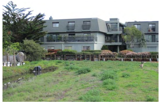
Condos along Saltworks Canal, Strawberry. Credit: Marin County DPW
