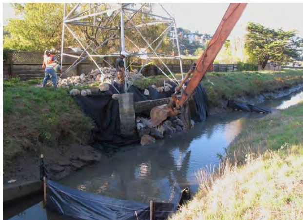
PG&E repair from storm damage in Tam Valley. Credit: Marin DPW
