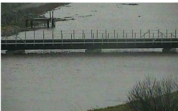
SMART Bridge, Novato. Credit: Marin County DPW
