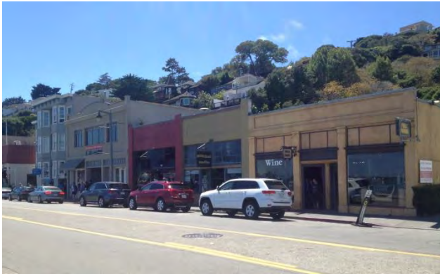
In the long-term flooding could impact Bridgeway and Downtown Historic District buildings lining its west side. Credit: Marin County CDA
