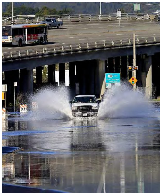
US Highway 101 on ramp at Manzanita is already flooded at high tides, especially combined with storms. Credit: Unknown
