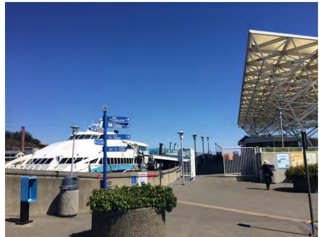
Golden Gate Ferry and Terminal. Credit: Marin County CDA
