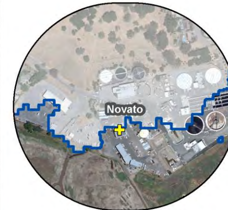
1: Novato Wastewater Treatment Plant
