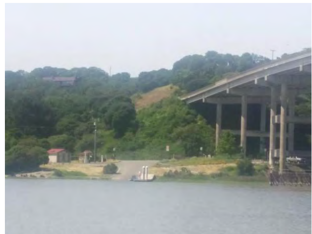
Black Point Boat Launch at State Route 37 and the Petaluma River. Credit: BYB Consulting LLC
