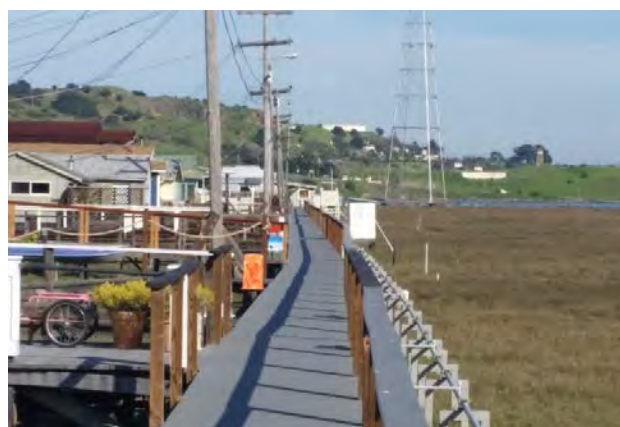
Greenbrae Boardwalk. Credit: BYB Consulting LLC
