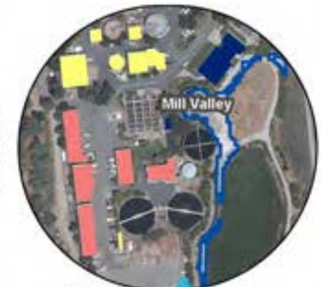
4: SASM Wastewater Treatment Plant
