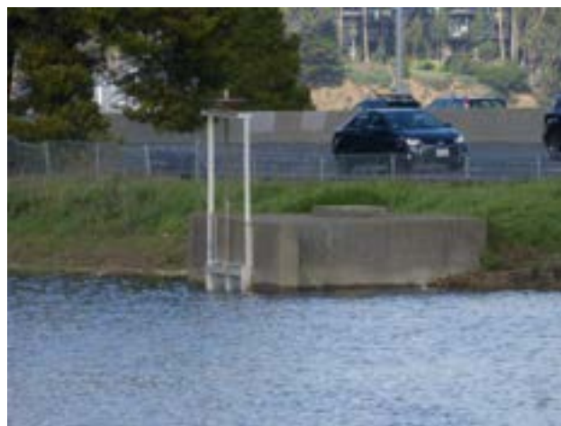
Stormwater Pond in Marin City. US Highway 101 is behind. Credit: Marin County DPW
