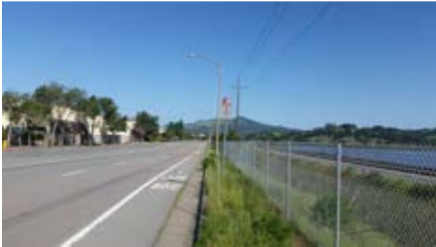
Rowland Blvd., bike lane, and SMART rail line behind the Vintage Oaks Shopping Center could be vulnerable. Credit: BVB Consulting LLC
