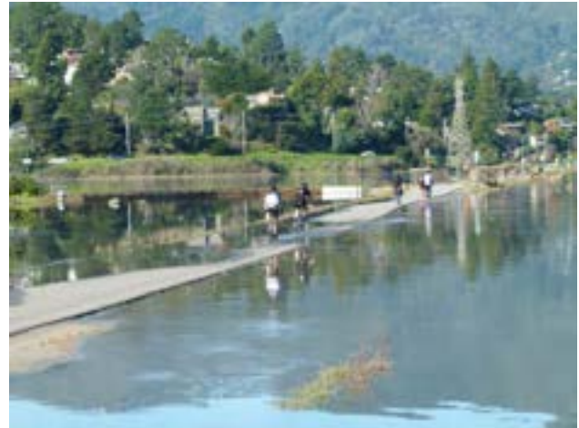
Bothin Marsh and the Mill Valley/ Sausalito Pathway Flooded at king tide. Credit: J. Poskazner
