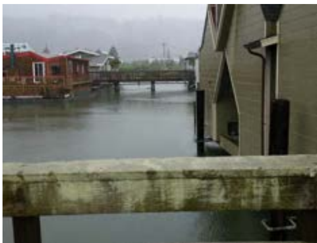
Richardson Bay Marina, East Pier 6 looking to the west pier. Waldo Point Harbor. April 2016. Credit: BVB Consulting LLC
