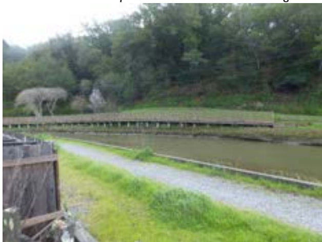
View of pathway and tidal zone of Coyote Creek. Tamalpais Valley. Feb. 2016. Credit: Marin County DPW
