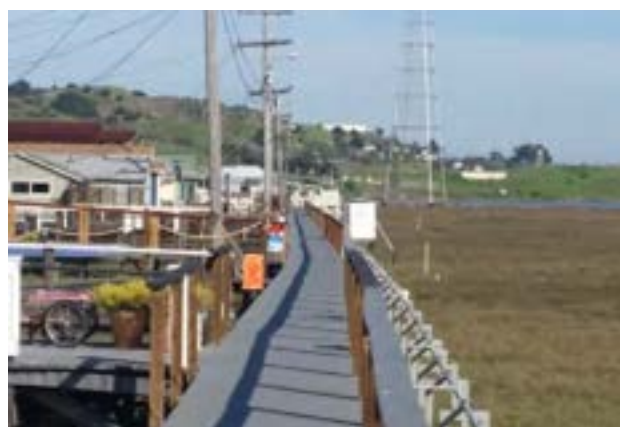
Greenbrae Boardwalk. Credit: BYB Consulting LLC
