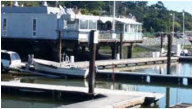
Loch Lomond Marina Club House. Credit: BYB Consulting LLC
