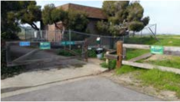
Stormwater pump station. Santa Venetia. Credit: BVB Consulting LLC
