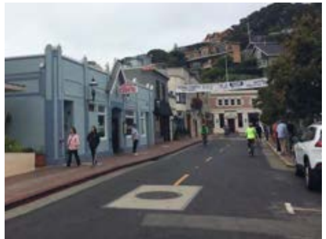
Tiburon's Main Street commercial buildings date back to the early 1900s, and are adjacent to the ferry terminal. Credit: Marin County CDA
