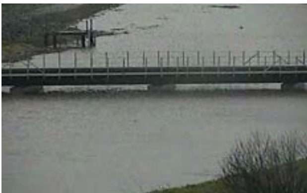
SMART Bridge, Novato. Credit: Marin County DPW
