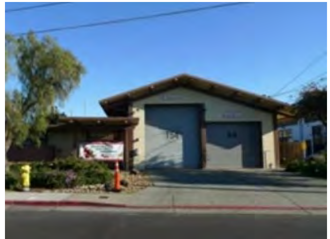
San Rafael Fire Station No. 54 is vulnerable. Credit: SRFD
