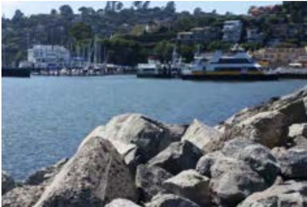
Tiburon revetment looking to Corinthian Marina and Tiburon Ferry Terminal, 2016. Credit: BVB Consulting LLC
