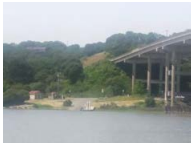
Black Point Boat Launch at State Route 37 and the Petaluma River. Credit: BYB Consulting LLC
