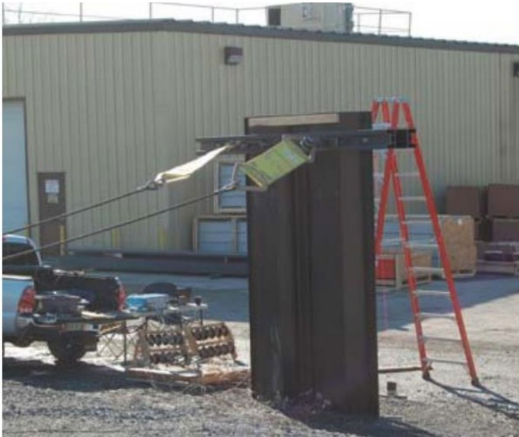
Figure 24 Sheet pile field test
