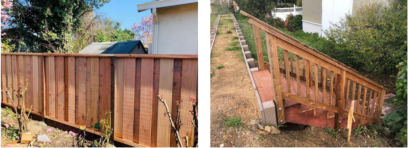
Figure 32 Fence and Staircase
