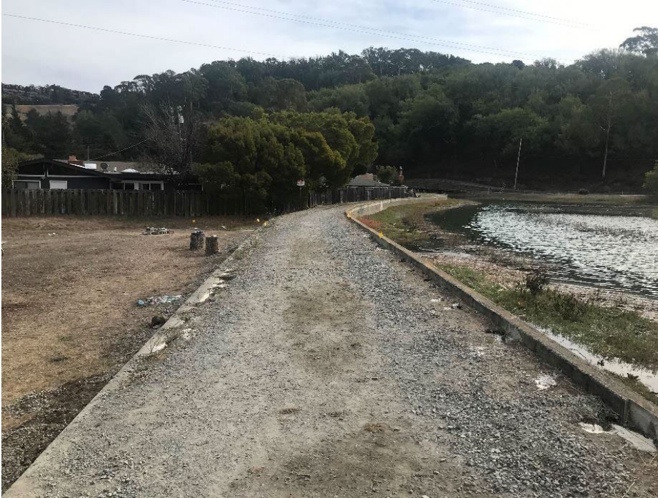
Levee adjacent to Flamingo Road
