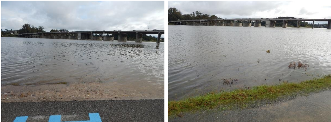
Photo 9. Shoulder of pedestrian/bike path berm along Richardson Bay, before complete submergence of paved path surface, one hour before extreme high tide of Jan 12, 2017.
