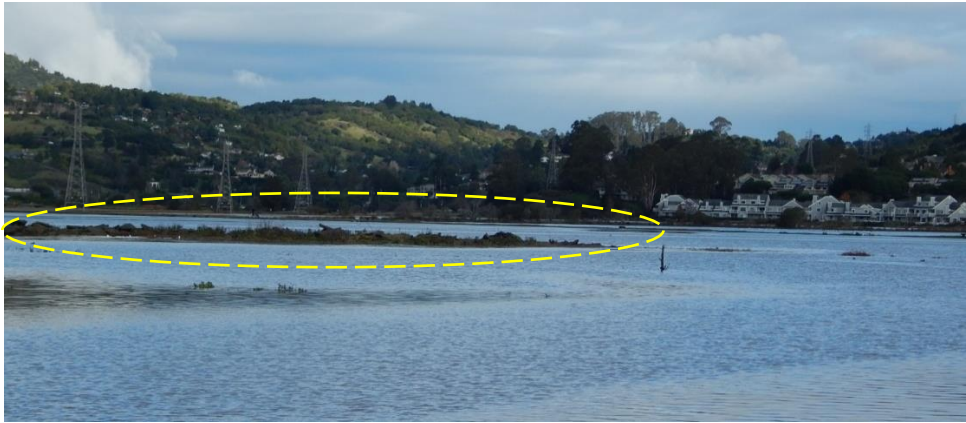
Photo 15. Island-like rubble debris pile above water level, South Bothin Marsh, 1 hour before extreme high tide January 12, 2017; high salt marsh and vegetation canopy is submerged.
