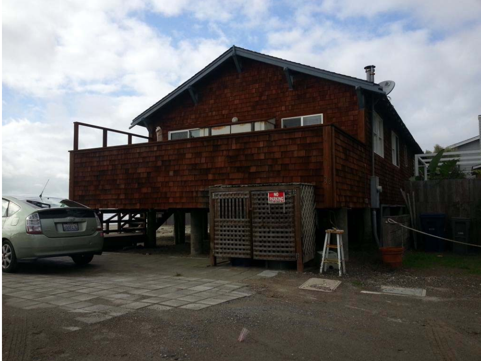
Figure 5.1 An Elevated House in the Study Area
