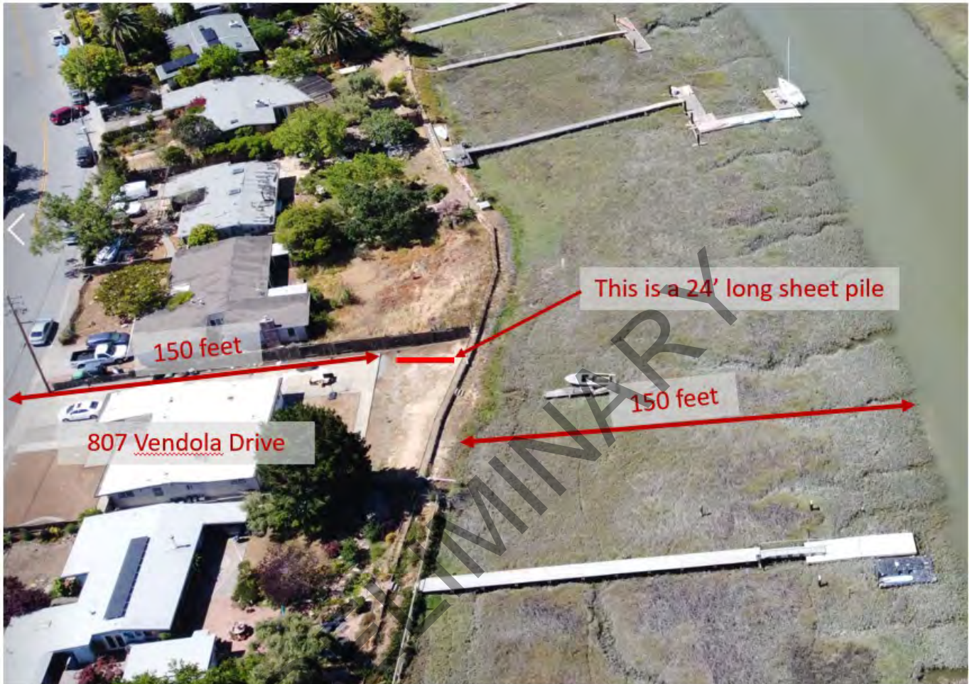
Figure 28 Land and water access to the work area
