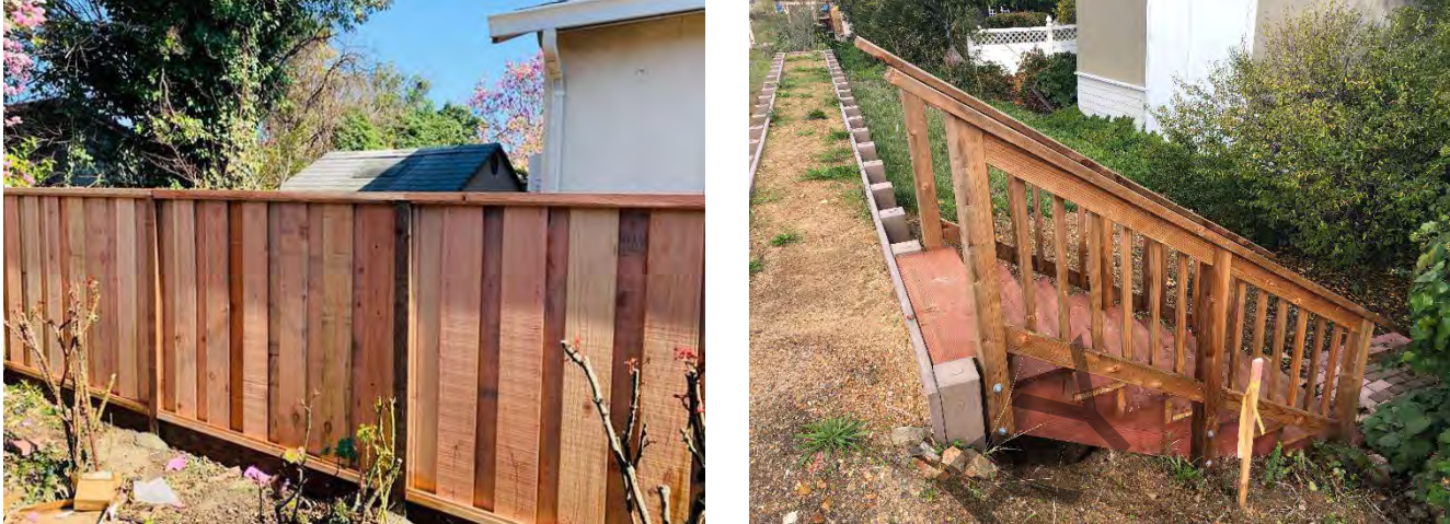
Figure 32 Fence and Staircase
