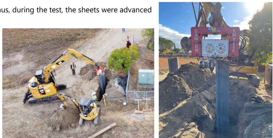
Figure 3. Sheet installation into trench.
