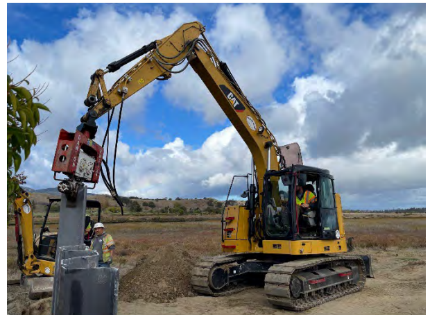
Figure 1. Sheet Pile Installation
