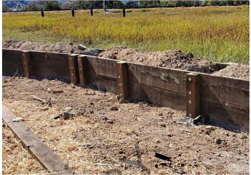
Figure 4 Example of a TRB installed at Santa Venetia
