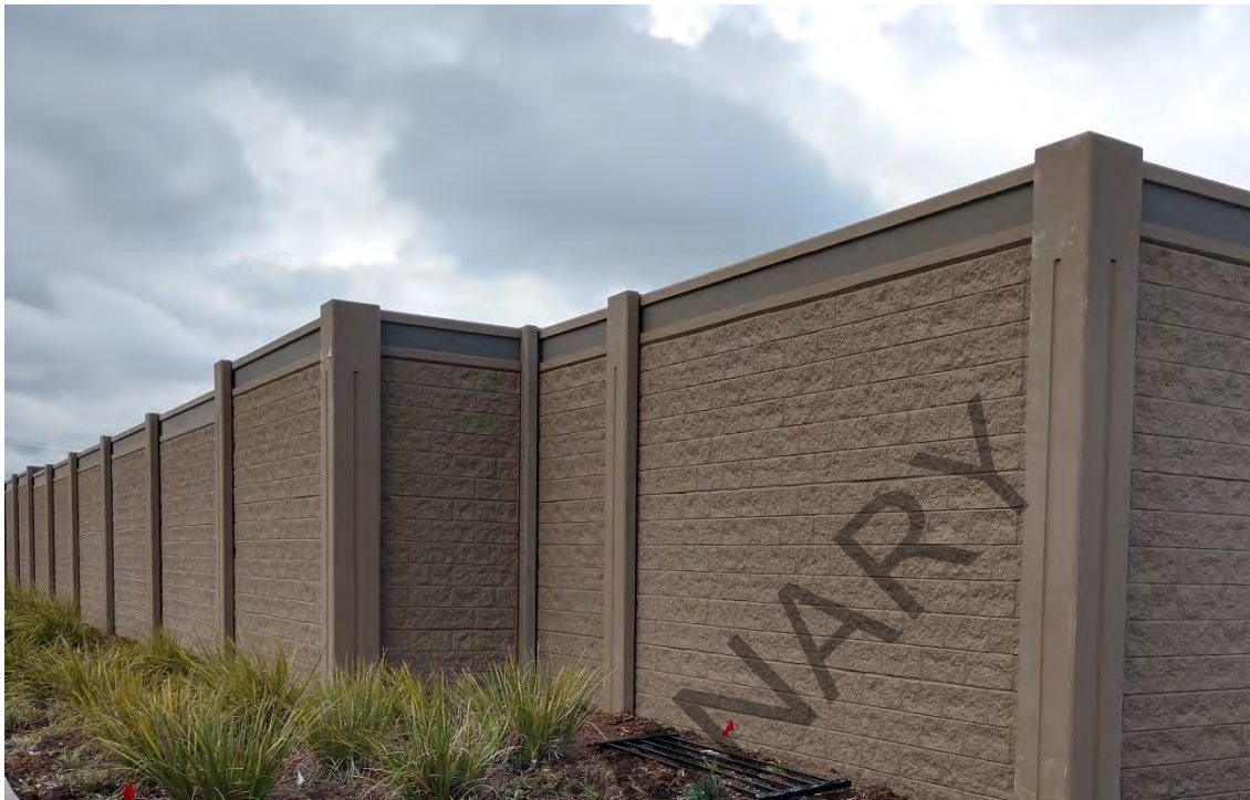
Figure 17 Precast Concrete Floodwall
