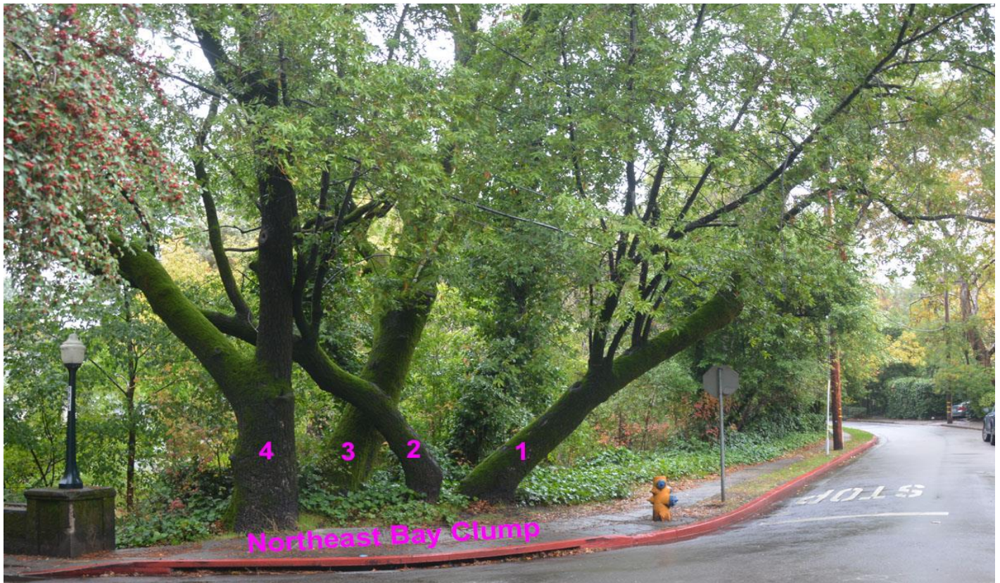
Figure 7 - Three of the four bays target the road or bridge and appear to have major structural defects. A full ISA Level 3 tree risk assessment should be done on these trees.
