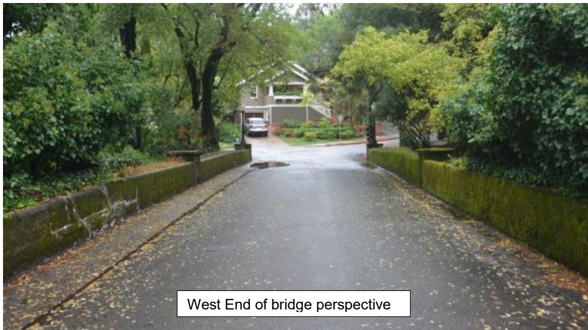
Figure 1 - The building opposite the east end of the bridge is the 33 Winship Avenue home.
