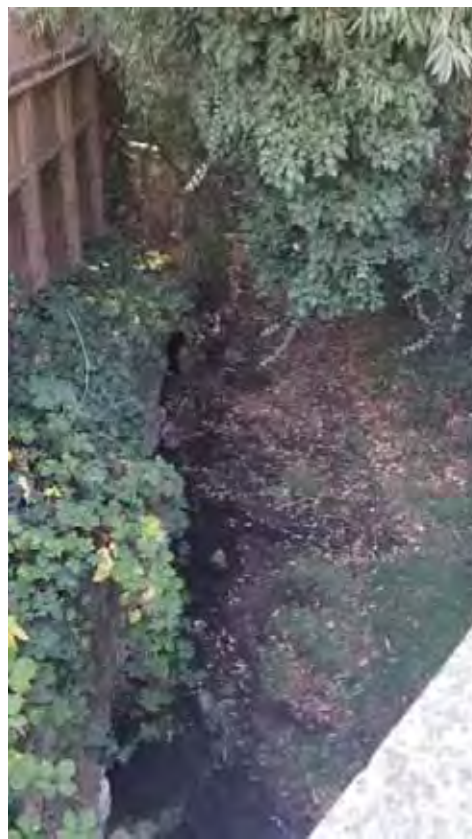
Figure A-7: Azalea Avenue Bridge Downstream Channel
