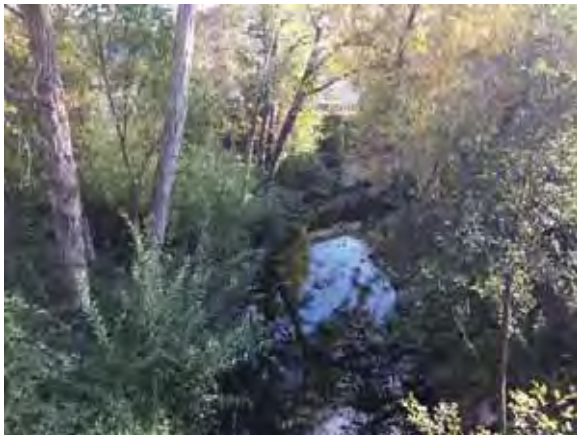
Figure A-13: View of Channel Downstream of Center Avenue Bridge
