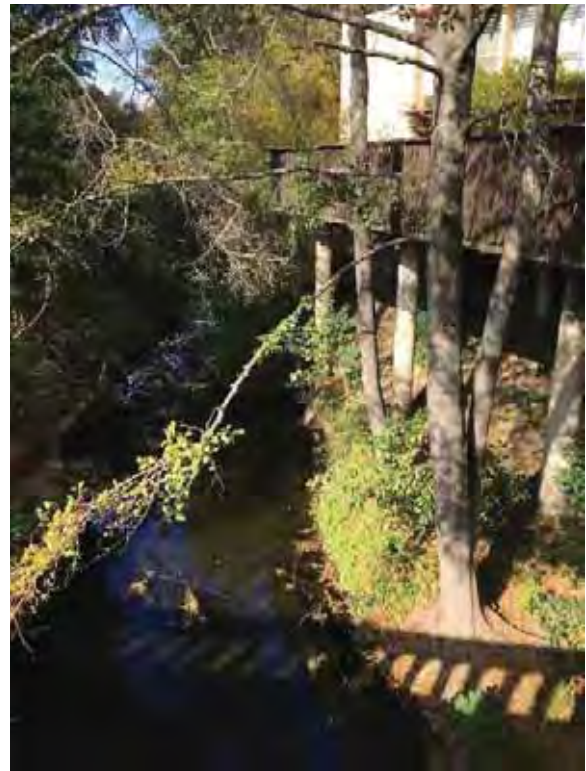
Figure A-14: View of Channel Upstream of Center Avenue Bridge
