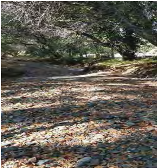
Figure A-1. Fairfax Creek Looking Upstream Looking along weir location showing active bank erosion and trees to be removed.
