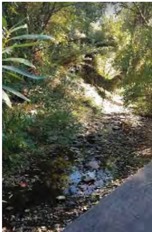
Figure A-5: Azalea Avenue Bridge Upstream View
