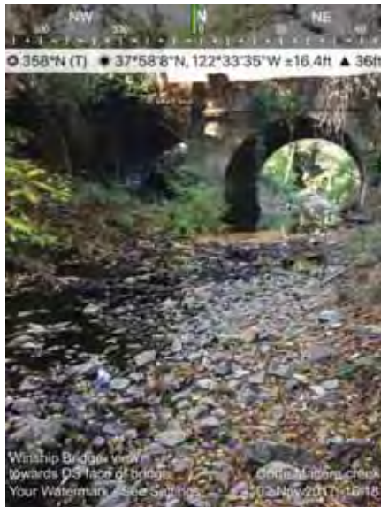
Figure A-18: Looking Upstream at Downstream Face of Winship Avenue Bridge
