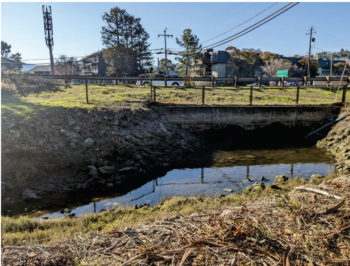
Photo 2. East Creek. Looking downstream from right bank of the grouted rock channel to the vertical concrete headwall inlet to the State Route 131 66" RCP "double-barrel" at Station 0+00' (December 16, 2022).
