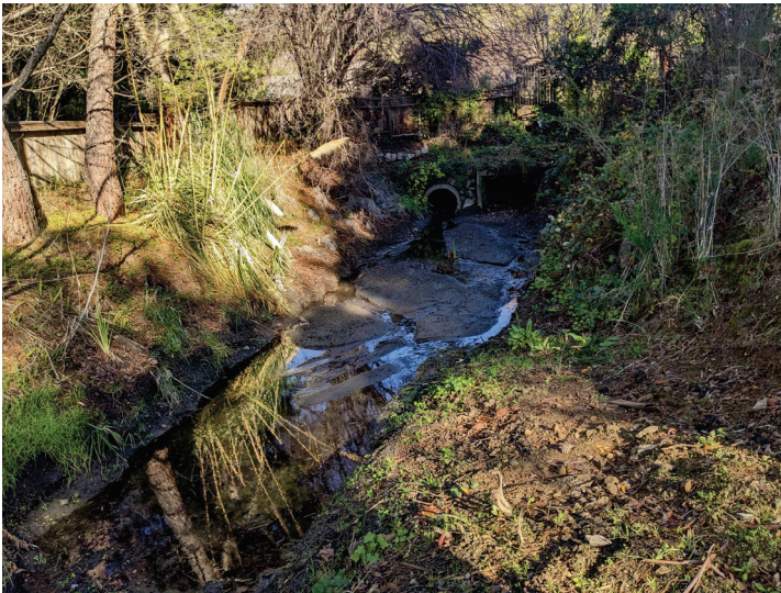
Photo 8. East Creek. Looking upstream to the outlet of culverts originating at or upstream from Karen Way (December 16, 2022). This is the maintained condition following channel maintenance dredging completed in October 2022. Note sedimentation near the culvert outfalls that occurred during November and December rainstorms.
