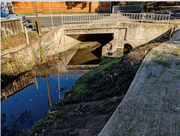
Photo 9. East Creek. Looking upstream to the outlet of Cecilia Way culvert (December 16, 2022). This is the maintained condition following channel maintenance dredging completed in October 2022. None or negligible sedimentation occurred downstream from Cecilia Way culvert during November and December rainstorms.
