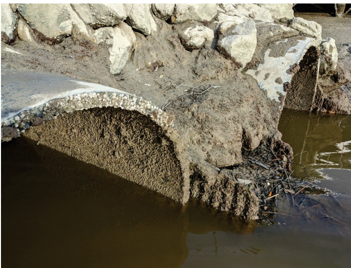
Photo 10. East Creek. View of the East Creek culvert outfalls in Richardson Bay near Station -3+95' (see also Photo 1). The original double-barrel 60" CMPs appear to have been slip-lined with 52" HDPE plastic pipe culverts (January 19, 2023).
