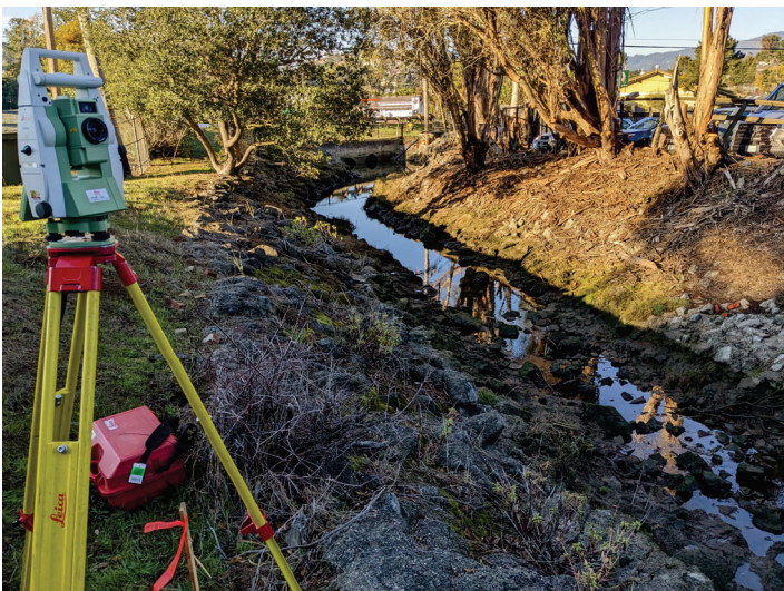
Photo 3. East Creek. Looking downstream from Control Point 1 near Station 1+55' to Lower East Creek. The grouted rock-lined channel extends from the sanitary sewer crossing near Station 1+80' to the State Route 131 "double-barrel" culverts headwall seen in background of view at Station 0+00' (December 16, 2022).
