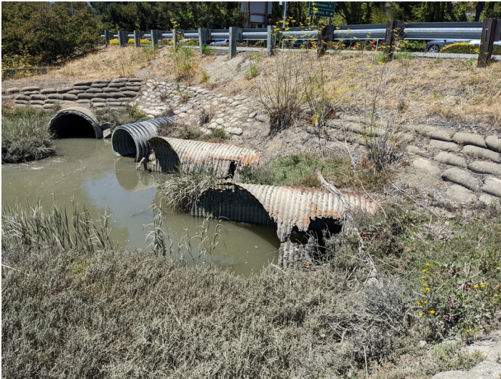
Photo 6. West Creek. Looking from left bank to outlet of two 60" CMP culverts (in foreground) outfalling to open natural channel downstream from Tiburon Boulevard (August 3, 2022).
