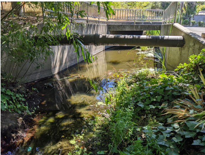
Photo 5. East Creek. Looking downstream from inlet to the 10-ft-wide open concrete box culvert and overhead sanitary sewer pipe crossing to 5'x10' Cecilia Way concrete box culvert downstream in background of view (August 3, 2022).
