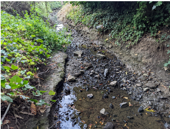
Photo 13. Lower West Creek. Looking downstream from the Lower West Creek channel bed near Station 4+10' to the lightweight foreign rubble deposited upstream from the rubble covered channel bed downstream, and evidence of recent natural tendency channel bed downcutting limited by coarse foreign material on the bed (August 17, 2022).
