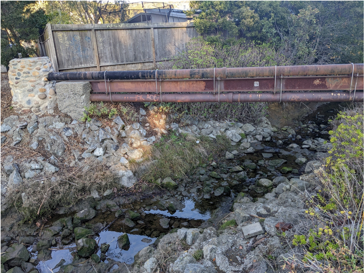
Looking upstream to East Creek from near STA 1+50' to RBSD sanitary sewer pipe crossing (December 16, 2022).
