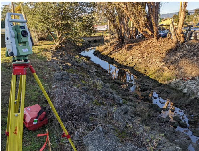
Photo 3. East Creek. Looking downstream from Control Point 1 near Station 1+55' to Lower East Creek. The grouted rock-lined channel extends from the sanitary sewer crossing near Station 1+80' to the State Route 131 "double-barrel" culverts headwall seen in background of view at Station 0+00' (December 16, 2022).
