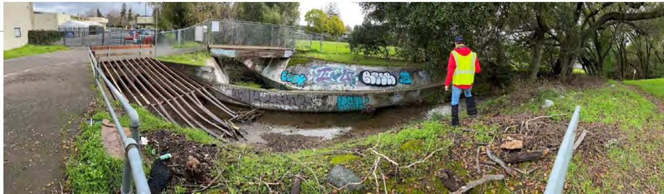
Existing Aroyo Avichi weir
