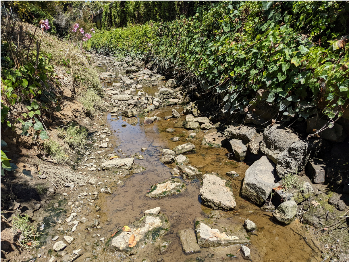
Looking upstream to Lower West Creek from near STA 3+30' (August 3, 2022).
