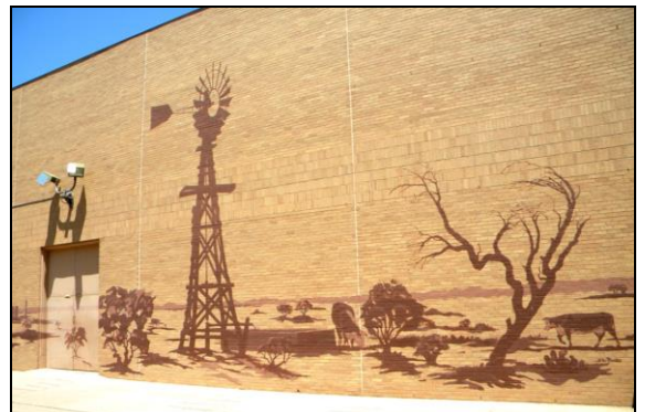
If painting on brick, do not paint the entire surface so that the brick can breathe. Midland, TX
