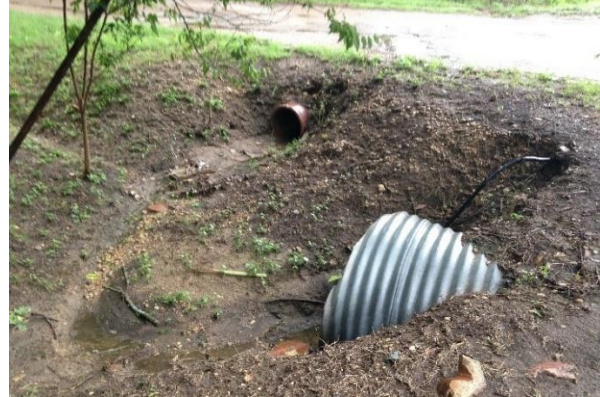
Figure 7E: Undamaged Culvert Example
