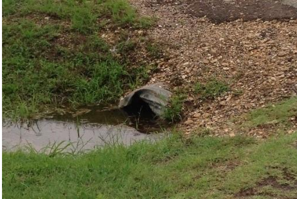
Figure 7D: Damaged Culvert Example
