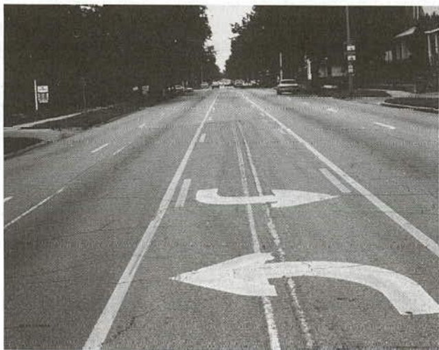
Figure 10. Example of incomplete removal of obsolete pavement markings which can create confusion to drivers on urban arterial streets
