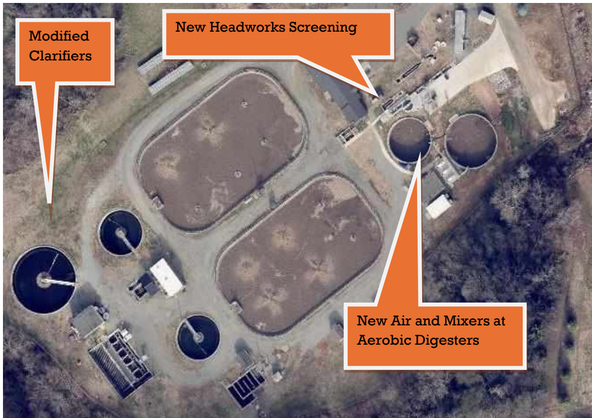
Figure 6. Renovated WRRF – Current
