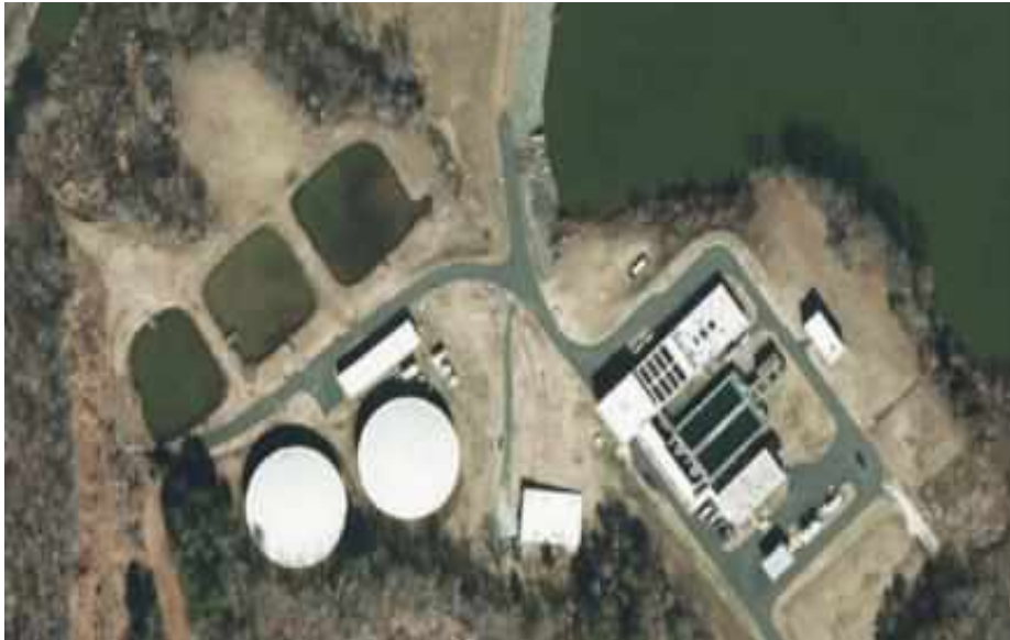
Figure 1. Graham-Mebane Water Treatment Plant 12.0 MGD
