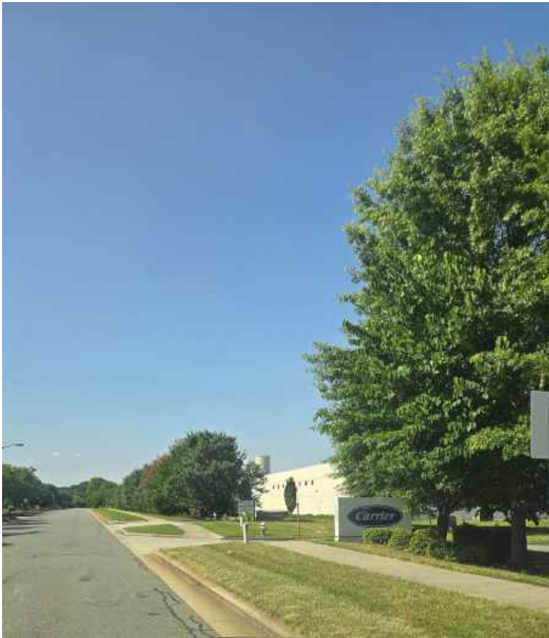
Photo 3 – Corporate Park Drive Looking South – 1,200 Feet
