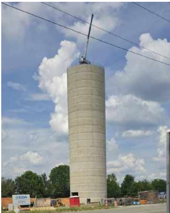
Figure 2. New 1-million-gallon Elevated Water Storage Tank is under construction.
