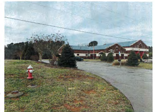
FIRE STATION 3 - MEBANE OAKS ROAD
