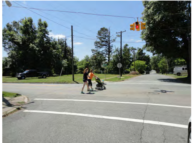
Pedestrians cross at Fifth Street and Jackson Street. While some crosswalks are present, they are missing for other legs.
