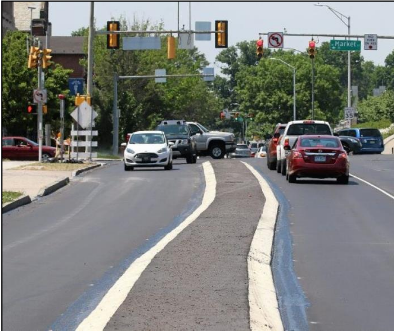
Figure 25: Example of a Mountable Concrete Median that could be installed on 5 th Street
