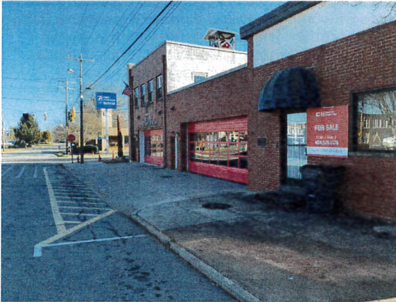
OLD FIRE STATION - DOWNTOWN
