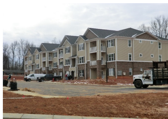
Soil Management at a Development Site
