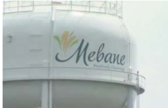
Mebane Water Tower
