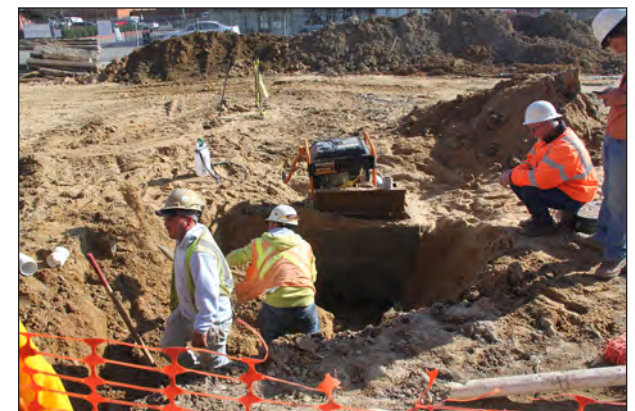
Infrastructure improvements in Goldsboro, NC.
