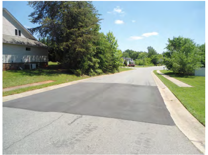
As the sidewalk changes sides of road, here at Fifth Street and Kit Street, there is no marked crosswalk connecting the two. This highlights a pedestrian crossing issue but can also be considered a gap to a connected pedestrian network.
