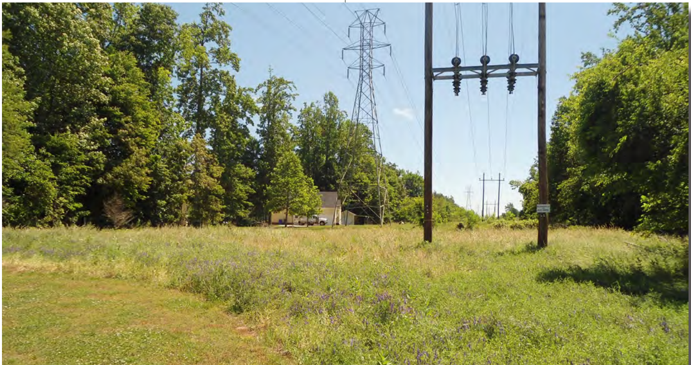
Power corridor near the Mebane Arts & Community Center soccer fields
