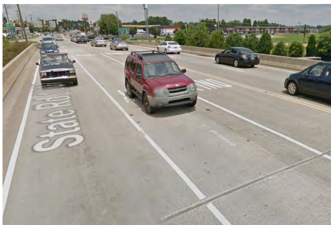
With approximately 1.5 foot paved shoulder across I-40 on Mebane Oaks Road, there is virtually no safe place for walking and bicycling.
