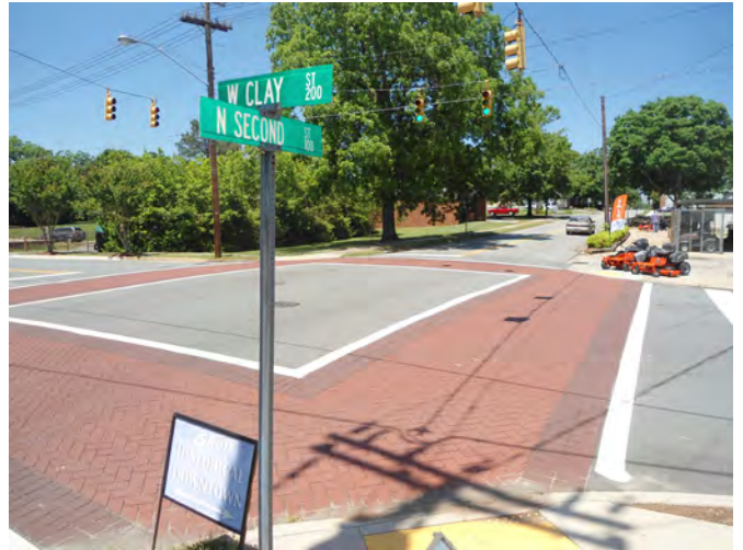
Clay Street marked crosswalks with pavers are high-quality and high-visibility in the Downtown core.
