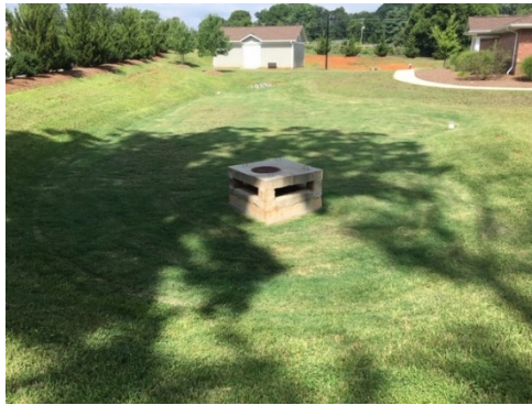
Bioretention Cell @ Mebane Ridge Assisted Living
