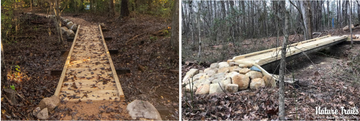
Examples of puncheon boardwalk with mud sills and 20ft clear span bridge from Nature Trails previous projects.
