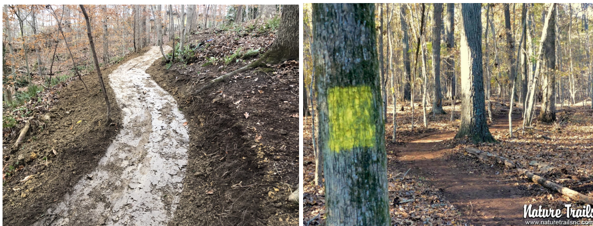
Example of bench cut and flat single-track trail from Nature Trails previous projects.
