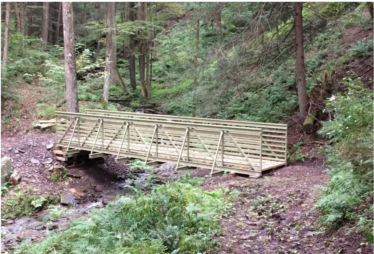
Example of Fiber Reinforced Plastic (FRP) bridge as recommended for any clear span over 30ft.
