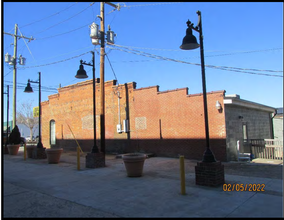
View of southern end of Buildings looking northwest
