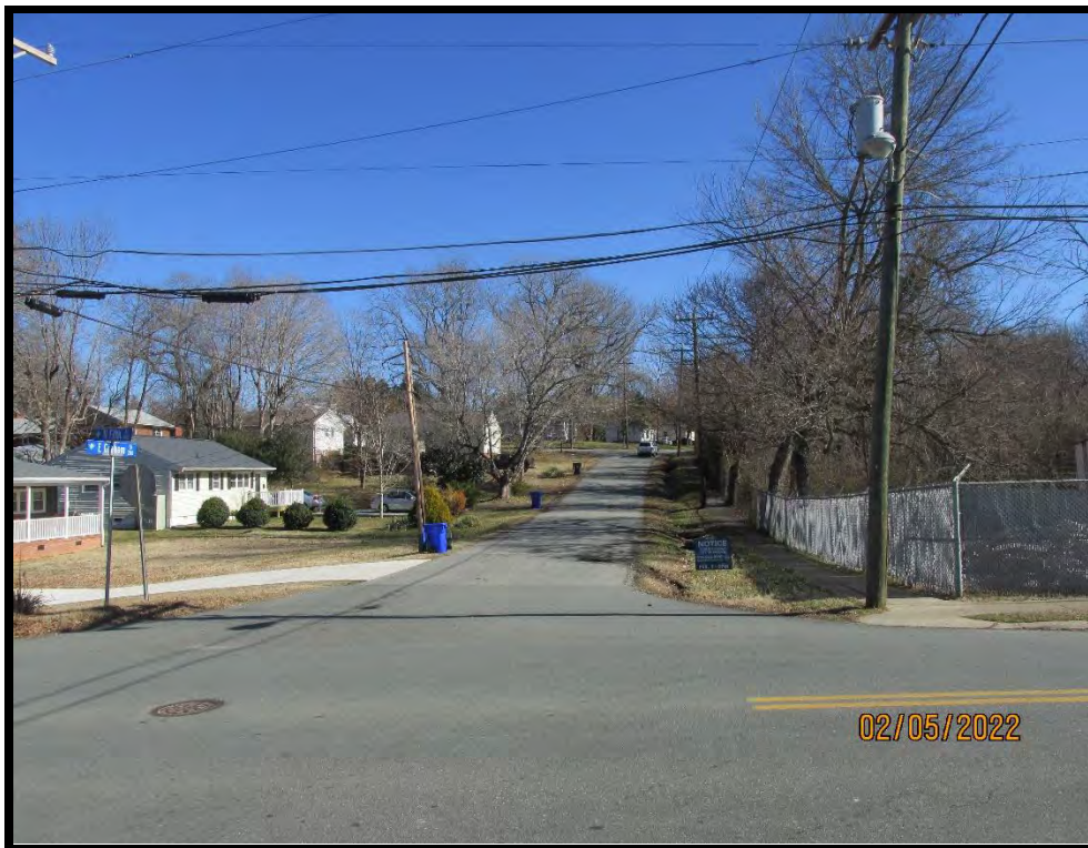
View of Graham Street looking east from N Fifth Street
