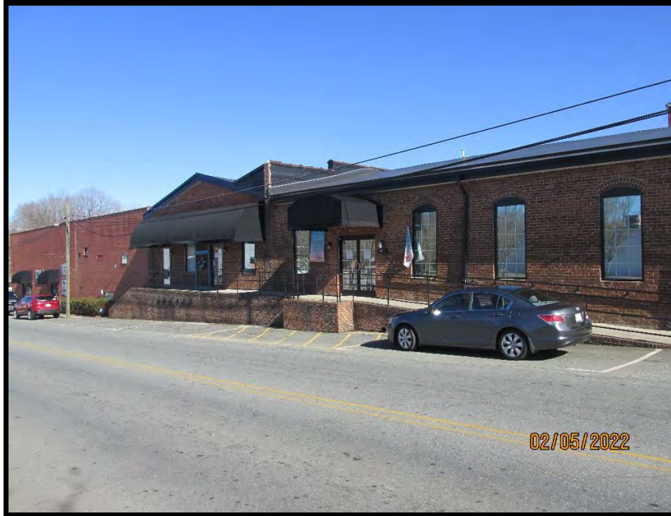
Front View of western side of existing Buildings Looking Northeast
