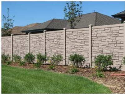
a. Masonry or Stone Wall
