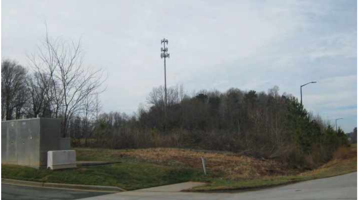
Tower near Collington
