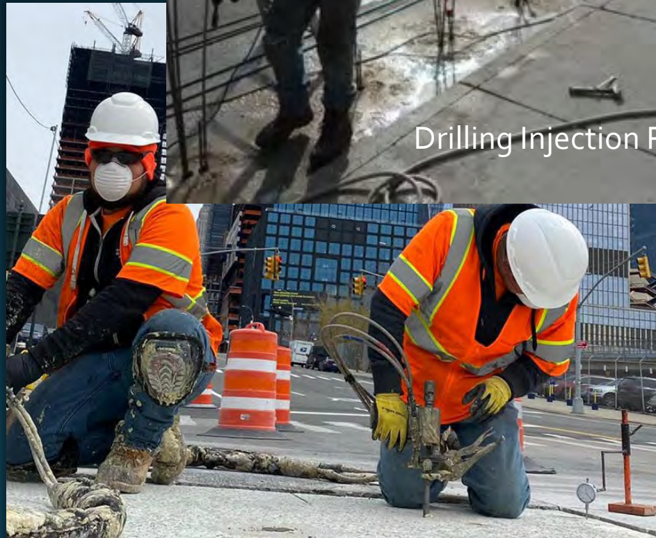
Drilling Injection Points
