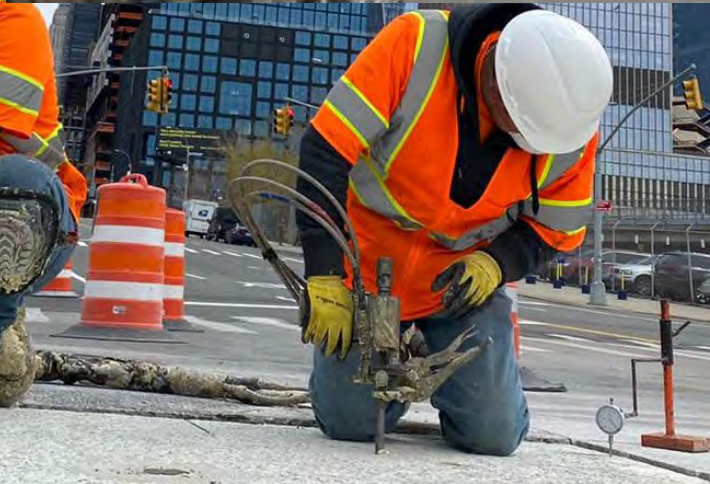
Drilling Injection Points
