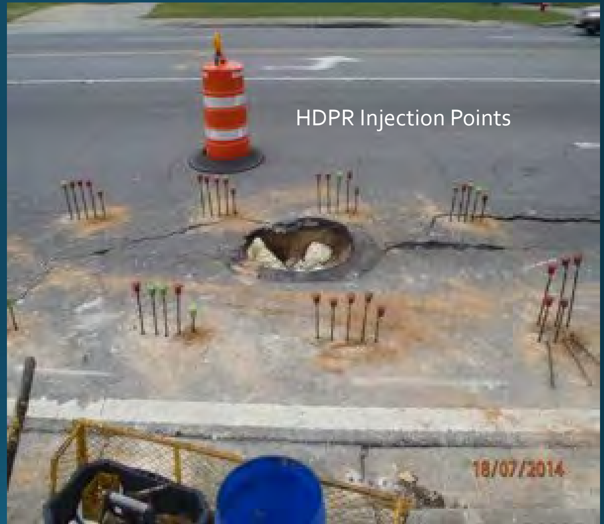
Drilling Injection Points
