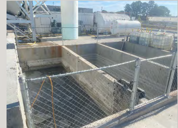
Sample Photos of Truck Washout and Sediment Bays
