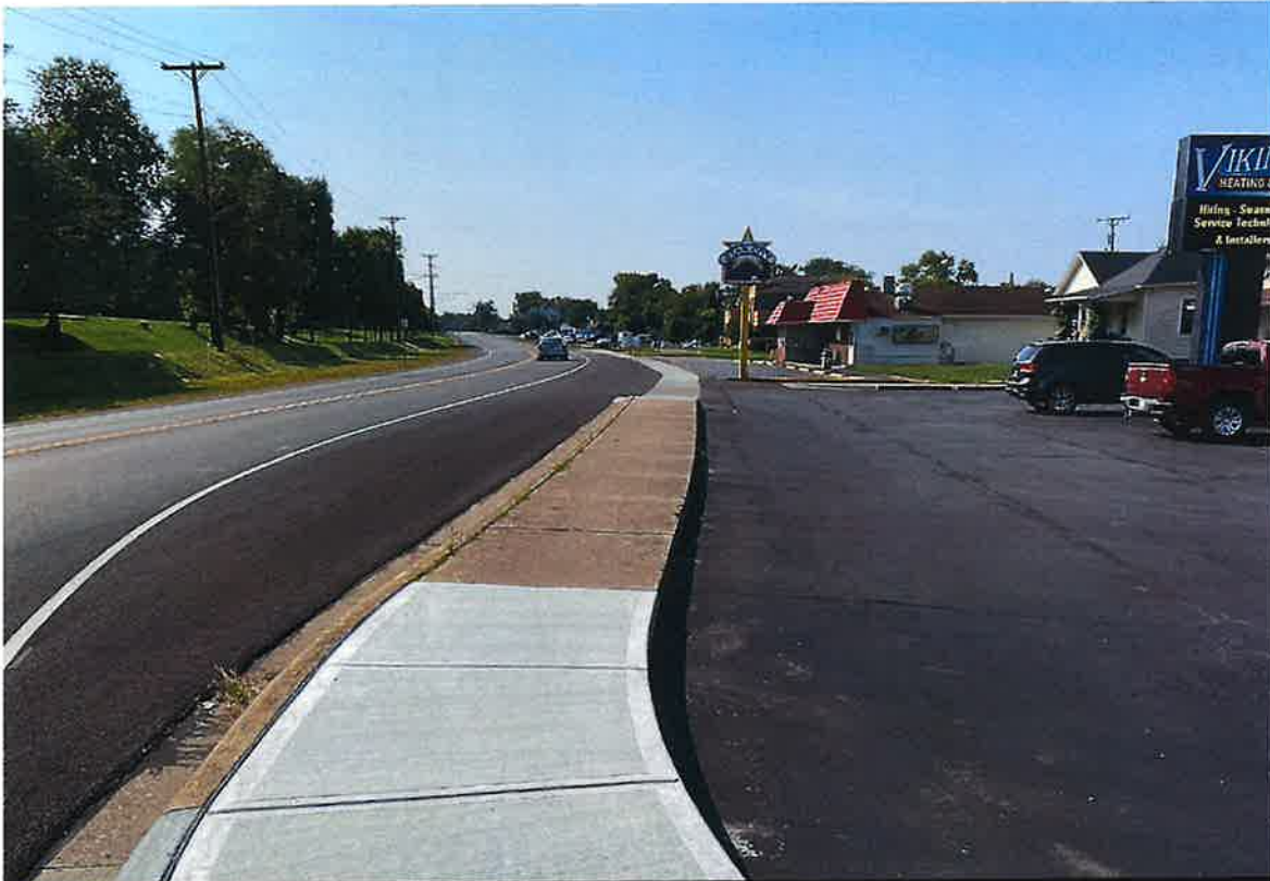
VIEW ALONG S. MAIN STREET (FACING SOUTH)
