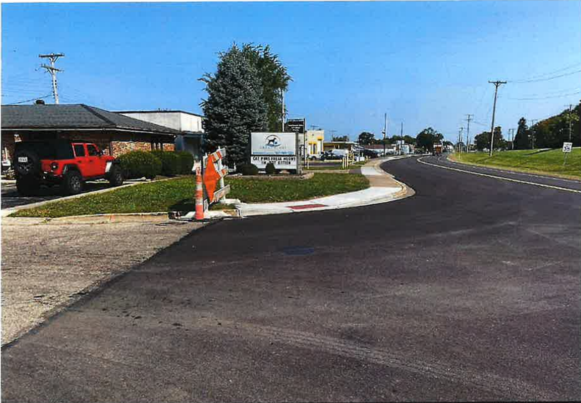
VIEW ALONG S. MAIN STREET (FACING NORTH)
