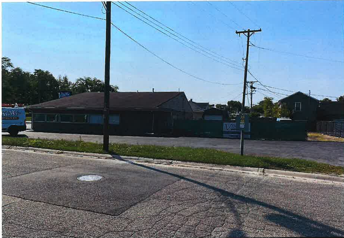
VIEW OF BUILDING FROM SOUTH STREET
